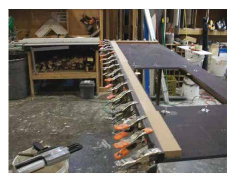
Attach the edge with 10 cm spring clamps (Pony spring clamps are fine), one every 10 cm, and leave until the adhesive is dry (about 1 hour).
