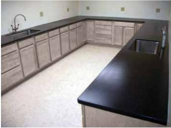
Kitchen and bathroom worktops must always be treated with Osmo® TopOil. The treatment must be carried out with a double application on the top, bottom and edge of the countertop.
